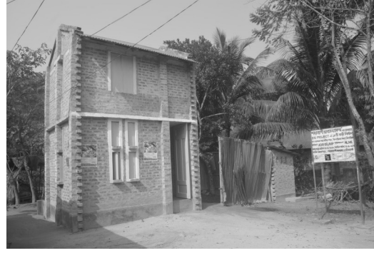
Figure 5: A two storied house in Vennatola (Co.Creation.Architects, 2018)
