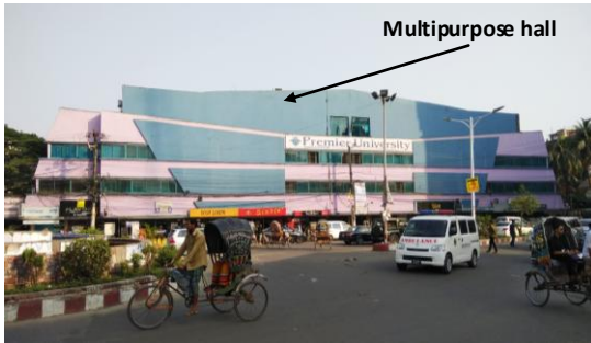
Figure 3: Premier University (PU) with surrounding context.
