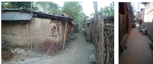
Figure 3: Decay of untreated mud and bamboo (left) result popularity for brick and cement construction (right)
