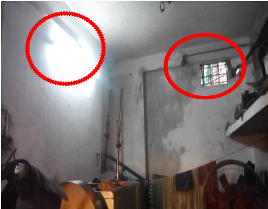
Figure 6: Workers resting space. Source: Author
