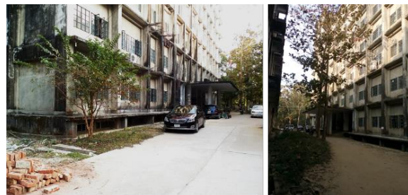
Figure 10: View of the building
