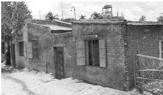
Figure 1: The picture shows a Transformed House in Mirpur, Bangladesh: This house was bought in 1980 for Tk. 5,500 and it was extended in 1988 at a cost of Tk. 60,000 (eight months' income). There were four households and 18 occupants in 1999. (Source: Tipple, A. Graham 1999)
